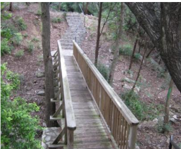
Pictures from the newly cleared trails around the tennis courts.
